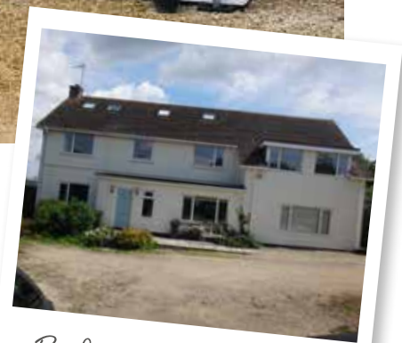
Before the renovation
