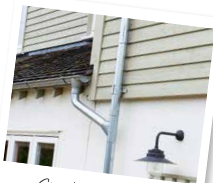
Steel guttering
